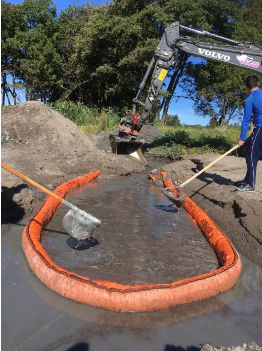
Figure 22. Removal of pellets using a net.
