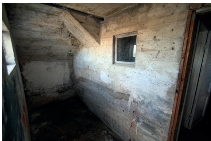
Under: Rom under trapp, rom 1-014.
