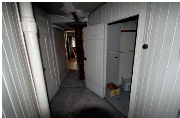
Over: Gang 1-211 sett mot gang 1-201. Under:
